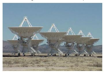
research facility that day. The VLA is a little-known New México treasure, and does research into all parts of space. It consists of 21 large parabolic antennas that can be moved along double railroad tracks.
